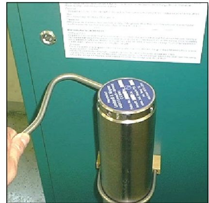
Fig. 1 - Unscrew the filter housing cover.
