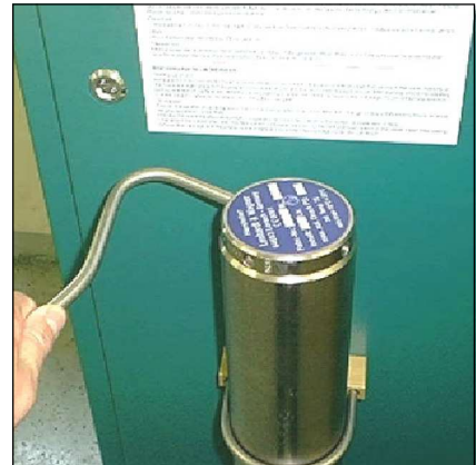
Fig. 1 - Unscrew the filter housing cover.
