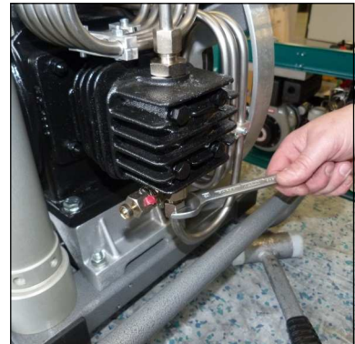
Fig. 1 - Loosen pipe connections
