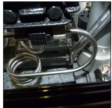
Fig. 2 - Loosen pipe connections of the filter housing
